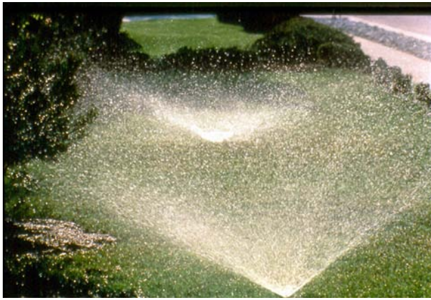
Figure 1. Fixed spray heads typically used to irrigate small or irregular landscape areas (Photo courtesy of Water Education Foundation).
